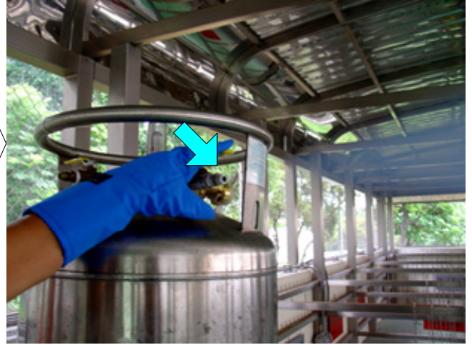
(4) Open venting valve till the pressure is less than 0.5 bar.
