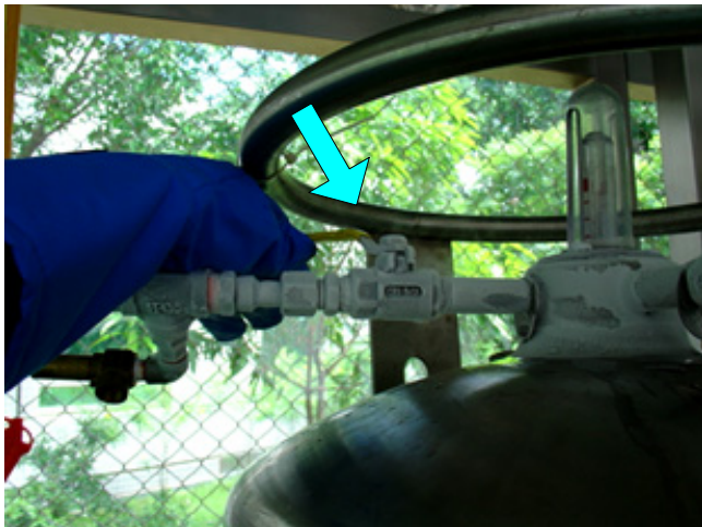
(2) When nitrogen exhaustion diminishes, close the refilling valve.
