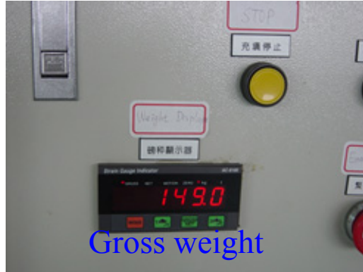
(5) Refill will stop at every 20KG increment. ( Refill will stop 10 seconds at every 90 seconds interval)
